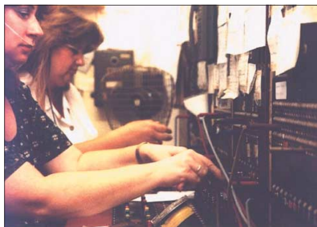
A hospital switchboard in 1995—shows the operators' directory and temporary notes. With permission from Martin Loach
